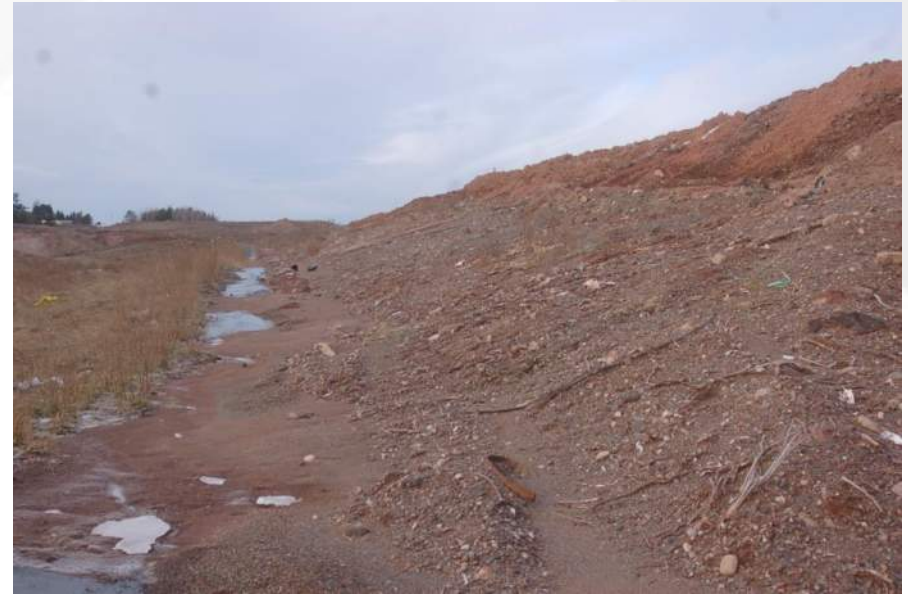
Photo 12 - Phase 3/4 South Working Face
