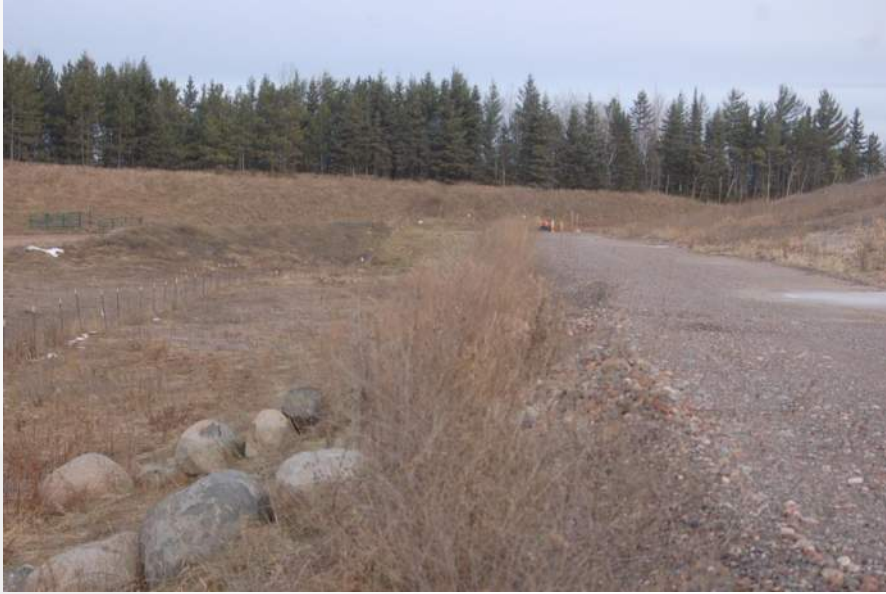
Photo 21 - Phase 2 Exterior Slope
