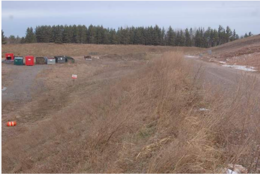
Photo 15 - Phase 2/3 Exterior Slope
