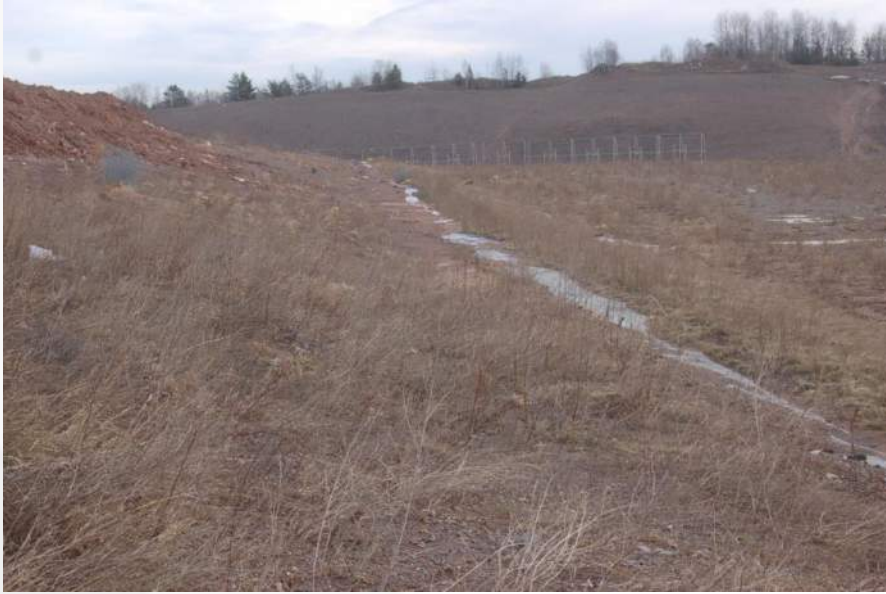
Photo 17 - Phase 4 South Toe/Waste Slope
