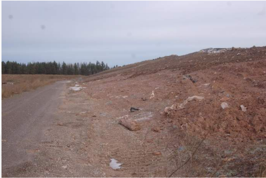
Photo 13 - Phase 2/3 West Waste Slope
