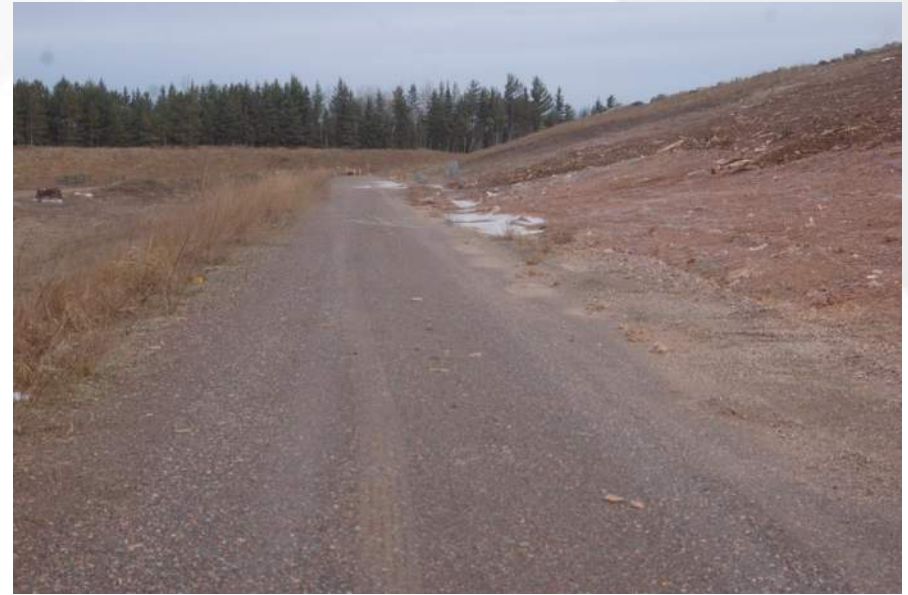
Photo 14 - Phase 2/3 Road/Toe Waste Slope
