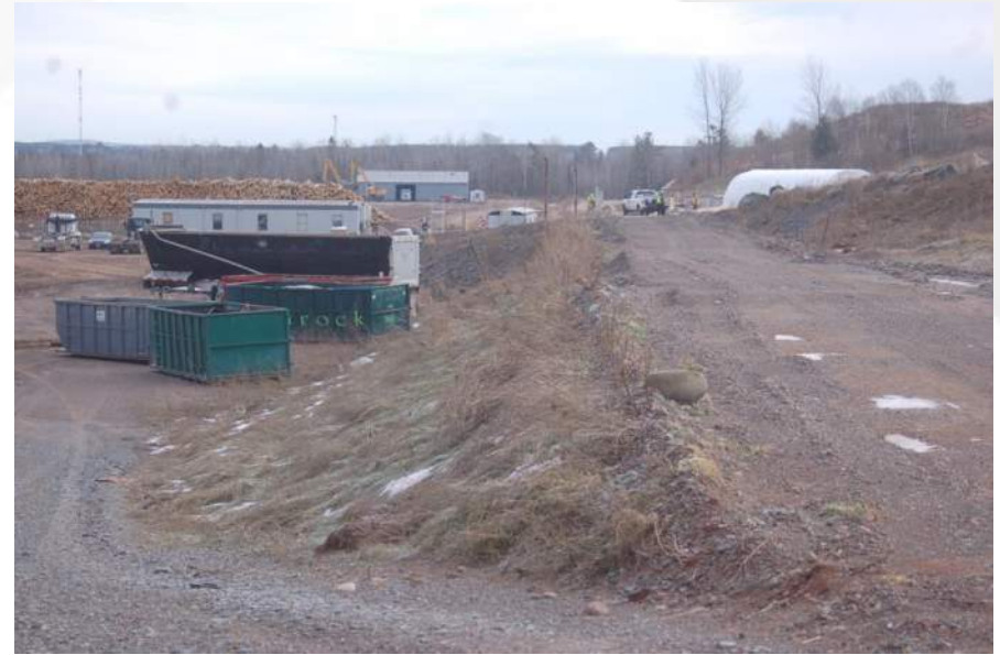
Photo 28 - Phase 2 Exterior Slope
