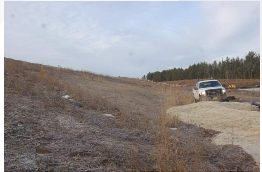
Photo 4 - Phase 1 and 2 North Slope
