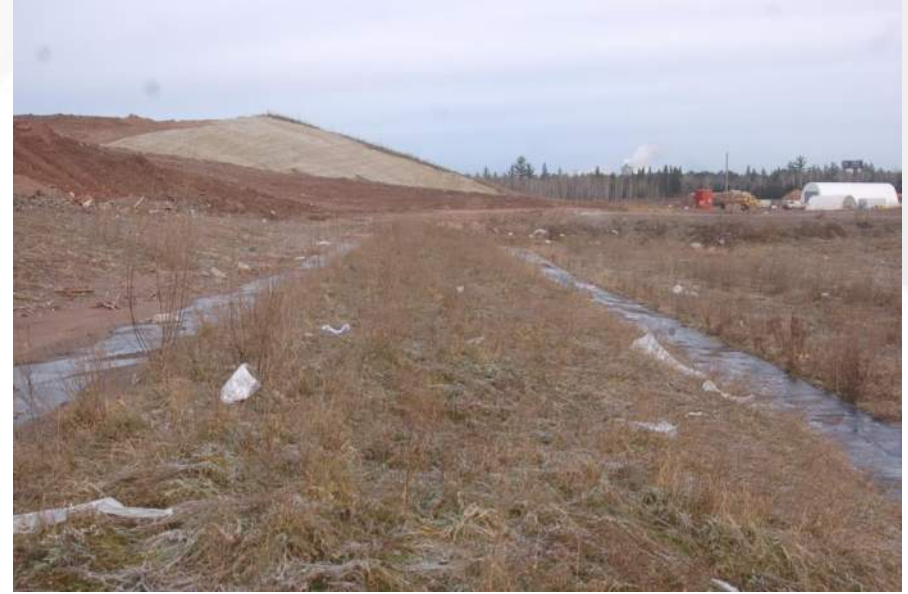
Photo 10 - Phase 4 East Working Face
