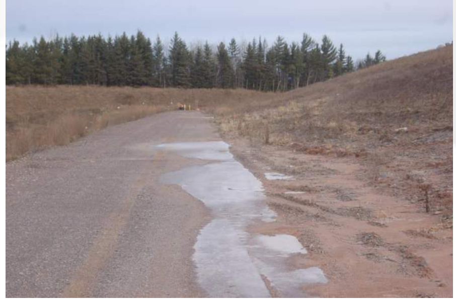
Photo 20 - Phase 2 West Road/Toe Waste Slope
