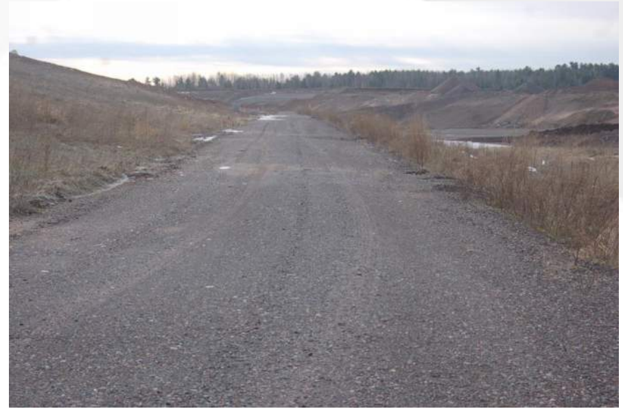
Photo 26 - Phase 2 Road/Toe/Waste Slope
