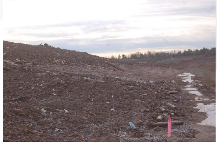
Photo 24 - Phase 3 Waste Slope
