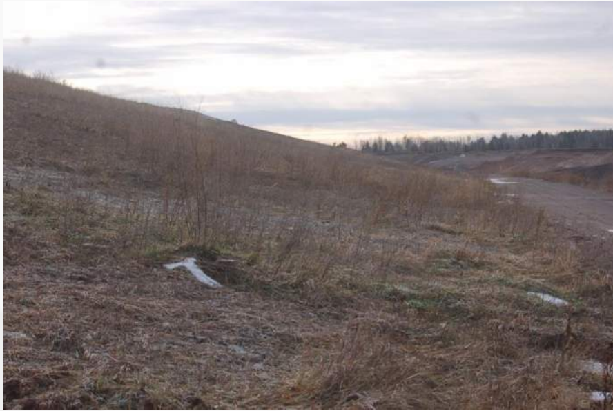
Photo 25 - Phase 2 Waste Slope
