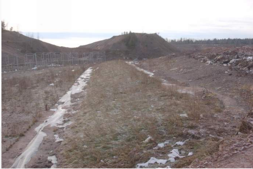
Photo 9 - Phase 4 East Exterior Slope
