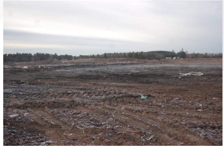
Photo 2 - Phase 3 and 4 Lower Active Area
