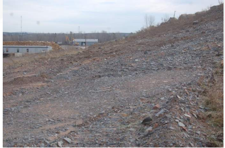
Photo 30 - Phase 2 Waste Slope
