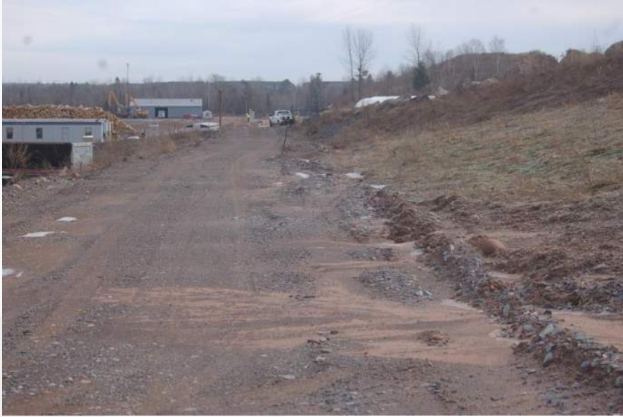
Photo 29 - Phase 2 Road/Toe/Waste Slope
